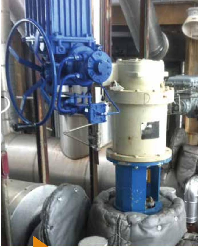
IM-15 WITH PNEUMATIC ACTUATOR IN SERVICE
